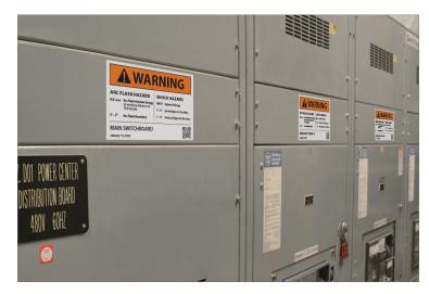
Figure 9.4: Example of Arc-Flash Labels Applied to a Distribution Board
